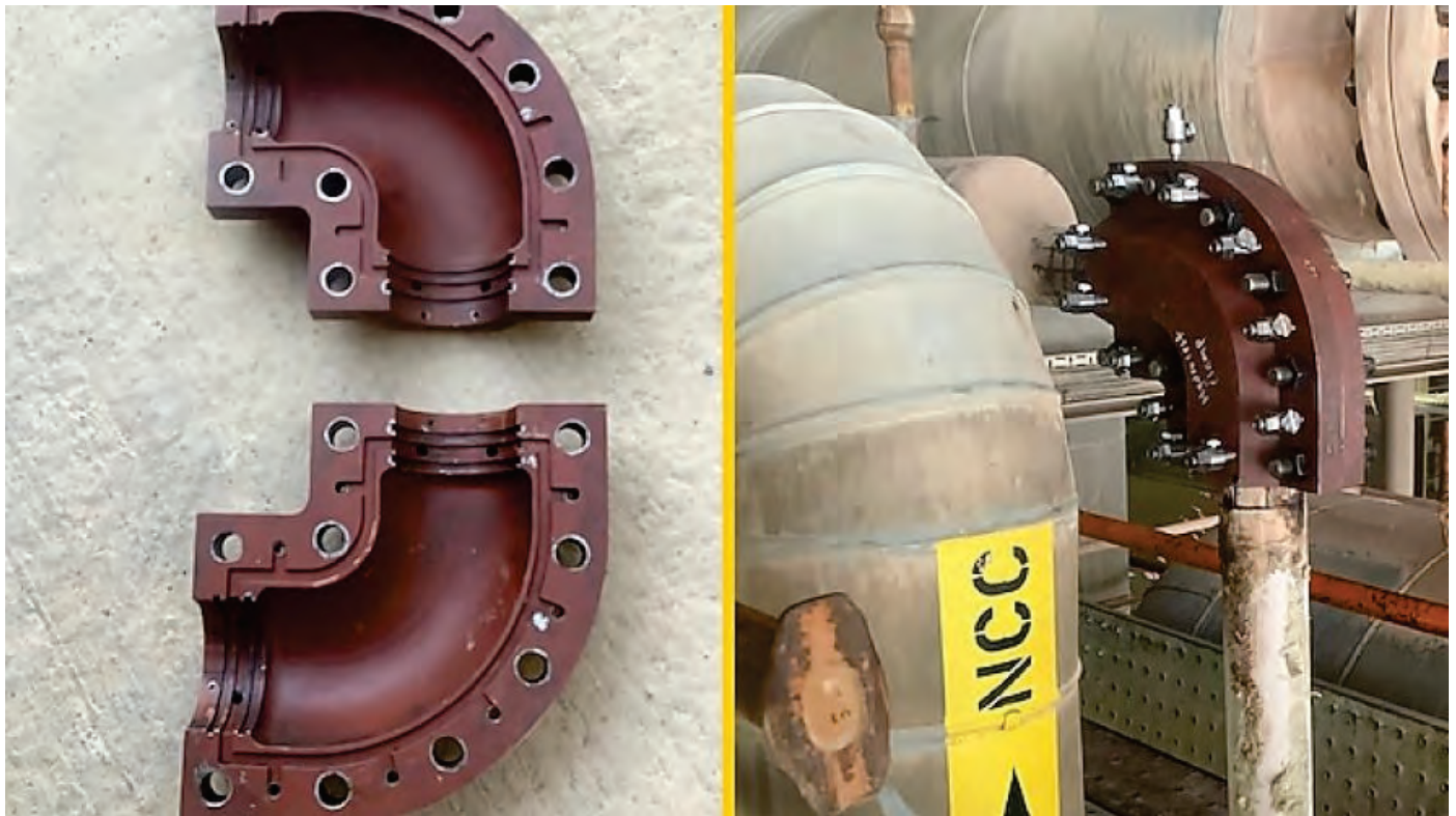
3D printed clamp installed at a Shell site
