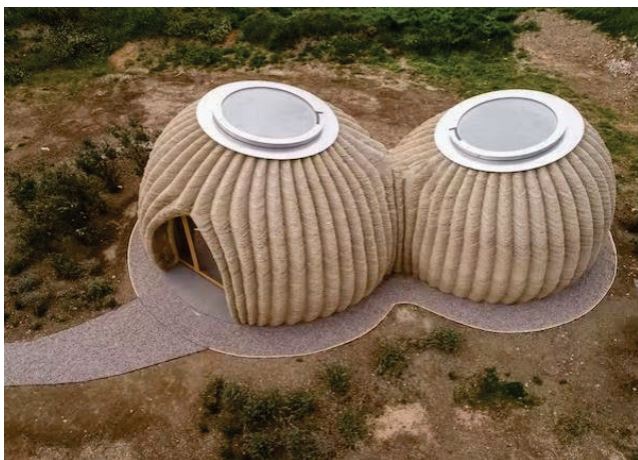
Tecla was built from locally sourced clay. Mario Cucinella Architects
