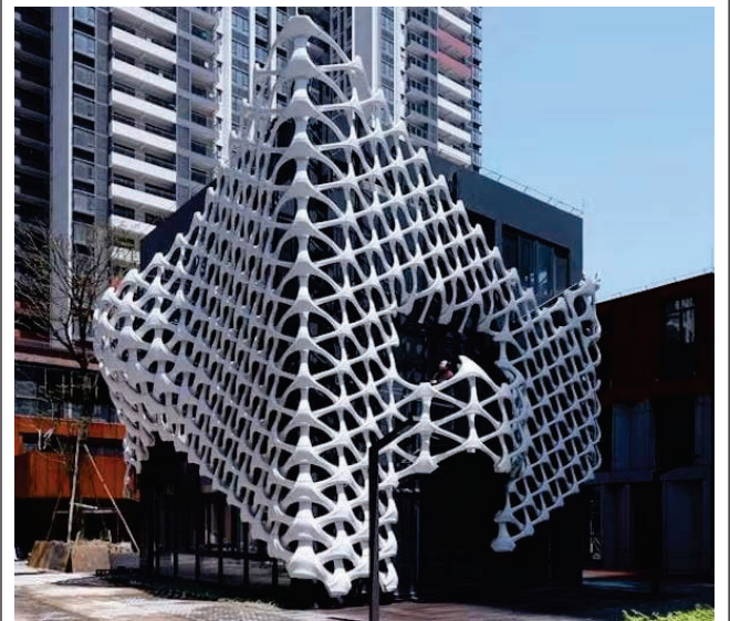
A 3D-printed façade in Foshan, China. The Association for Computer Aided Design in Architecture
