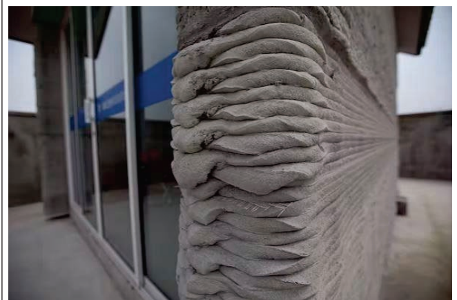
A 3D-printed house in Shanghai that was built in less than 24 hours out of construction waste. Visual China Group/Getty Images
