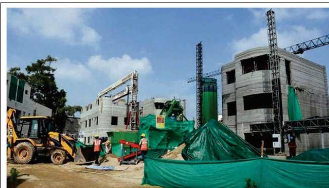
A complex under construction using 3D printing technology near Air Force Station, Behlana. NITIN MITTAL
